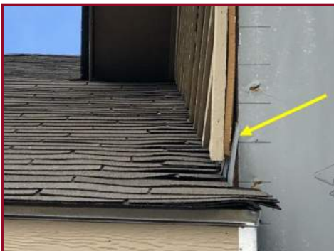
STEP FLASHING BEHIND EXTERIOR SHEATHING
