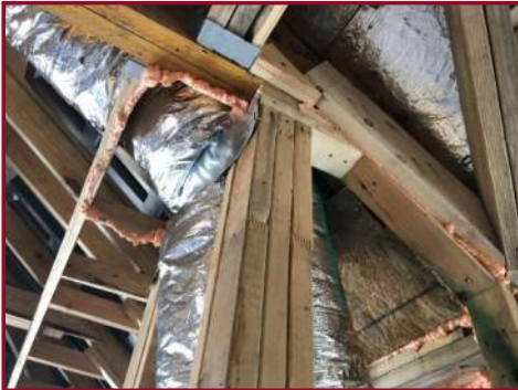
TRIPLE STUDS SUPPORTING INTERSECTION OF JOIST BEAMS AND ROOF RAFTERS
